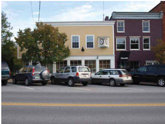
Example of 60 degree angle parking Manchester, VT
