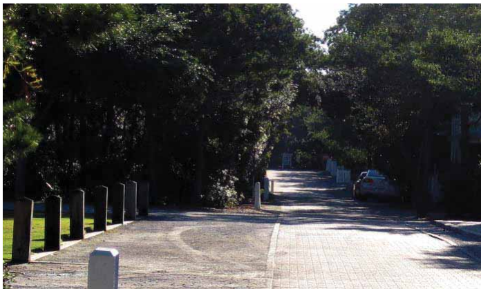
Example of crushed gravel parking area shown with narrow roadway of paver texture. Seaside, FL
