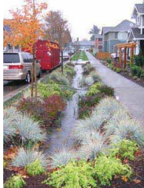
Example of a rain garden or bio swale Photo: Permission pending http://www.lakecountyil.gov Municipal Research and Services Center of Washington
