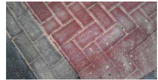
Example of applied polymer crosswalk shortly after completion Clarkstown, NY
