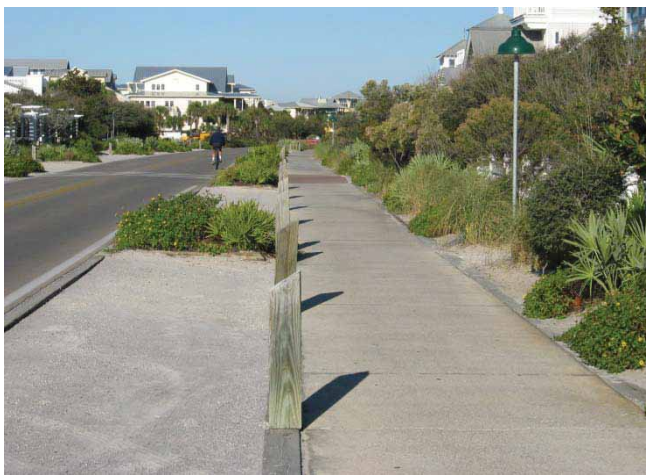
Example of a curbless separation between pedestrian and parking area - gravel parking area, concrete sidewalk Seaside, FL
