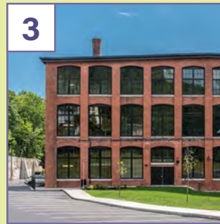
3 Yarn Works, Fitchburg, MA A former textile mill repurposed into apartments
