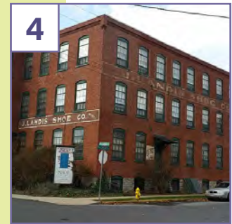
4 Shoe Factory Apartments Palmyra, PA A former shoe factory repurposed into apartments
